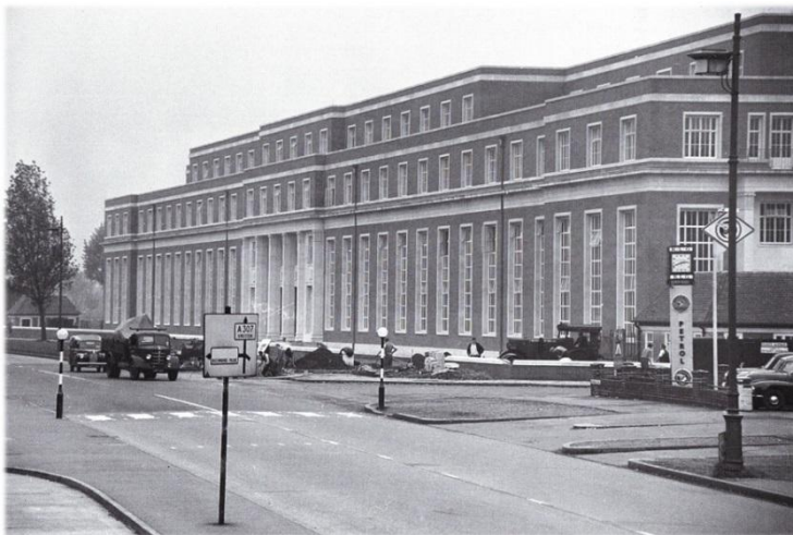
The Kingston factory (the Ham Works site) as it appeared after 1958 when a façade incorporating the new Head Office and Design Office had been completed.
